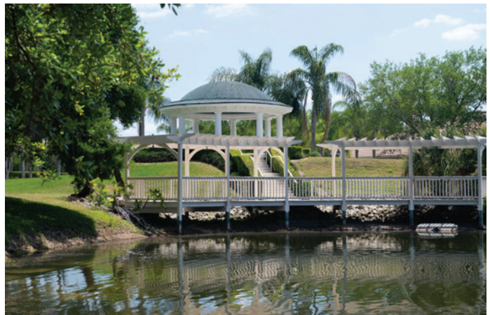
OBSERVATION DECK: Major repairs were made including repainting of the structure
