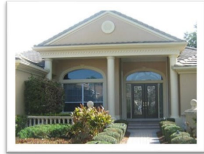
This home shows the relationship between the doors with inserts and side lights, the curved transom and the window to the side.
