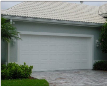
Garage door banded on 3 sides (note banded returns painted in trim color)
