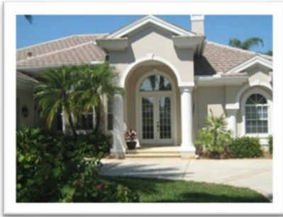
This home demonstrates the relationship among the doors with insert glass panes, the circle top transom and the window to the side.
